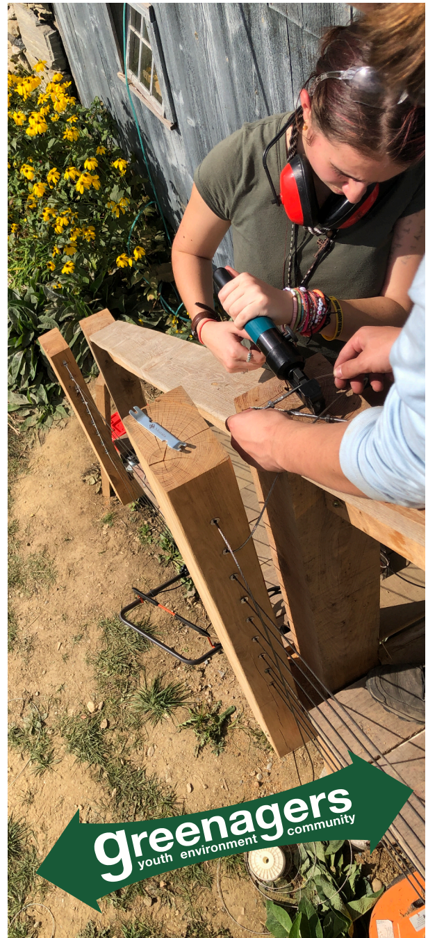
TRADES CREW BUILDING A NEW STAIRCASE ON THE BARN.
