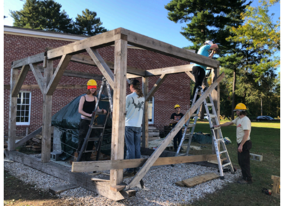
The Pathways team building a timber frame roof for the Sheffield Community Bread Oven.
