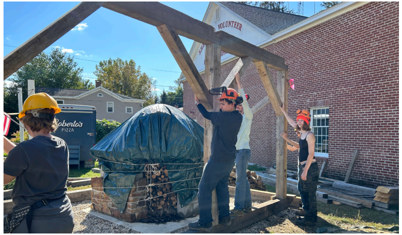
BUILDING A TIMBER FRAME ROOF FOR THE SHEFFIELD COMMUNITY BREAD OVEN
